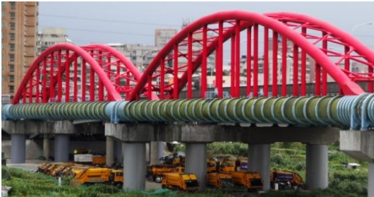
Yongfu arch water pipe bridge
