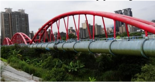
Hsintien arch water pipe bridge
