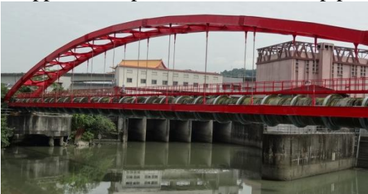
Yuanshan arch water pipe bridge
