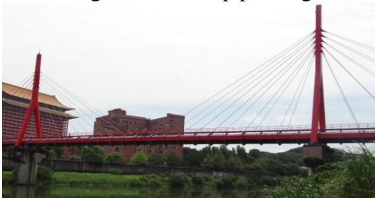
Jiantan cable-stayed water pipe bridge
